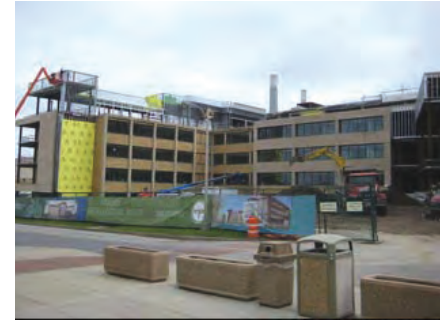
Renovations at Science Engineering and Technology SUNY Oswego
