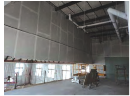
DOTY Building Renovation SUNY Geneseo
