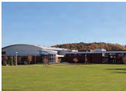
Jorgensen Center Rehab Mohawk Valley Community College
