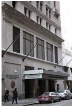
Exterior Renovation College of Optometry
