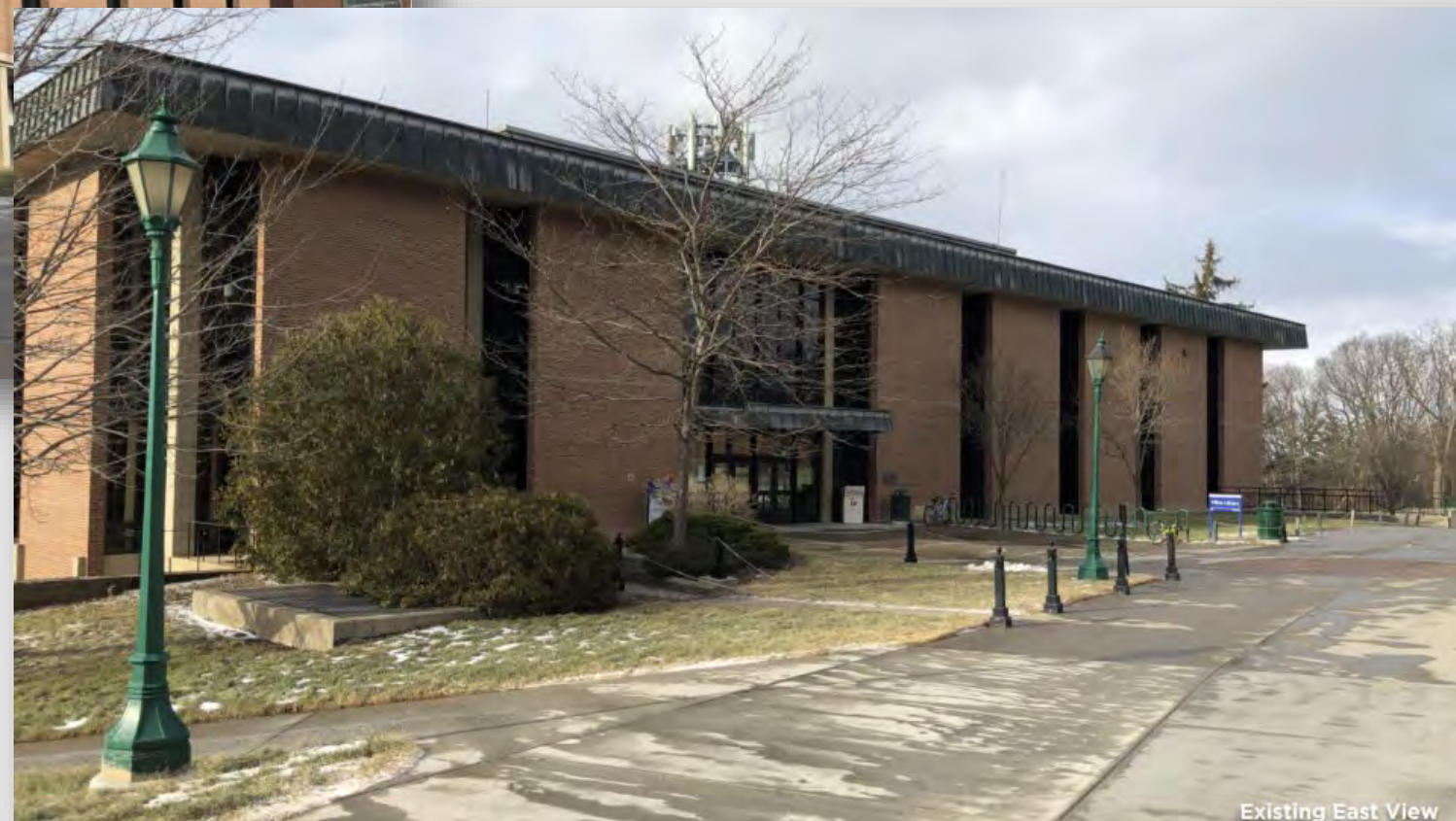
Existing East View
